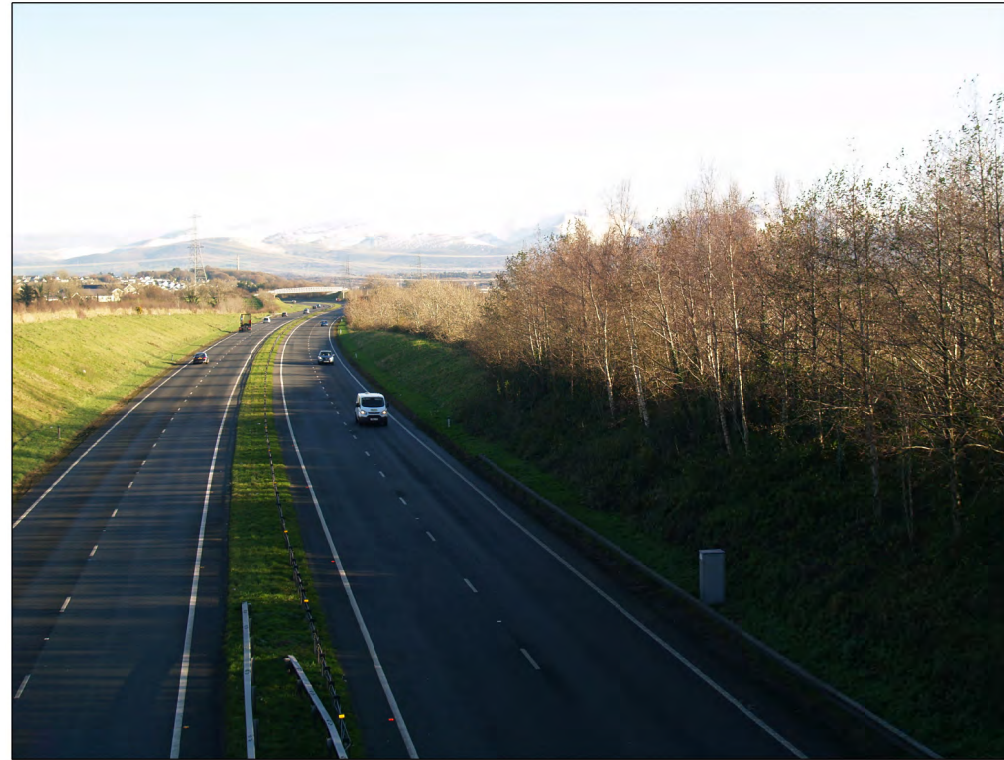
Photograph looking east over the A55. The site is in the middle distance on the right in the photograph
