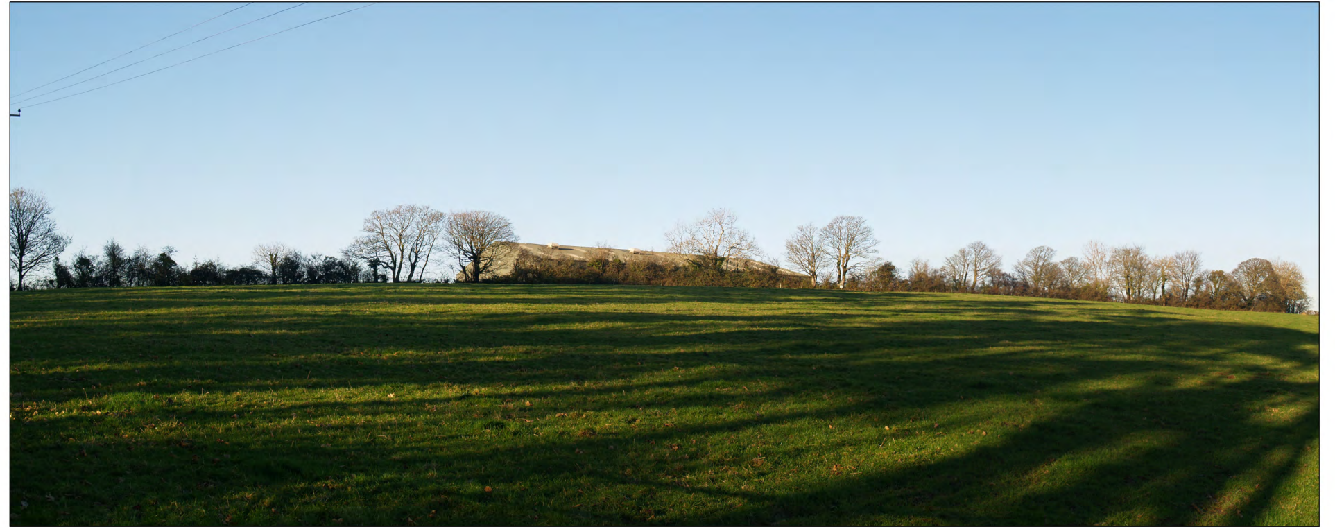
Photograph looking north towards waste transfer station from the site entrance access road
