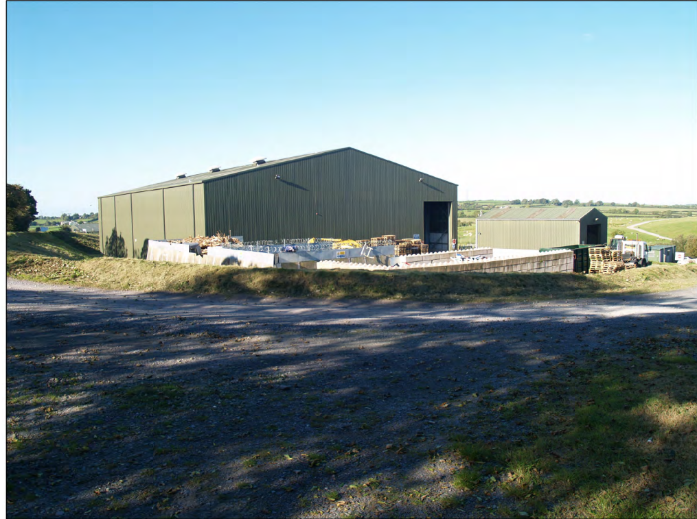
Photograph looking west towards the waste transfer station
